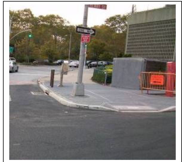
Newly installed pedestrian "bump-out" at Henry Street and Cadman Plaza.
